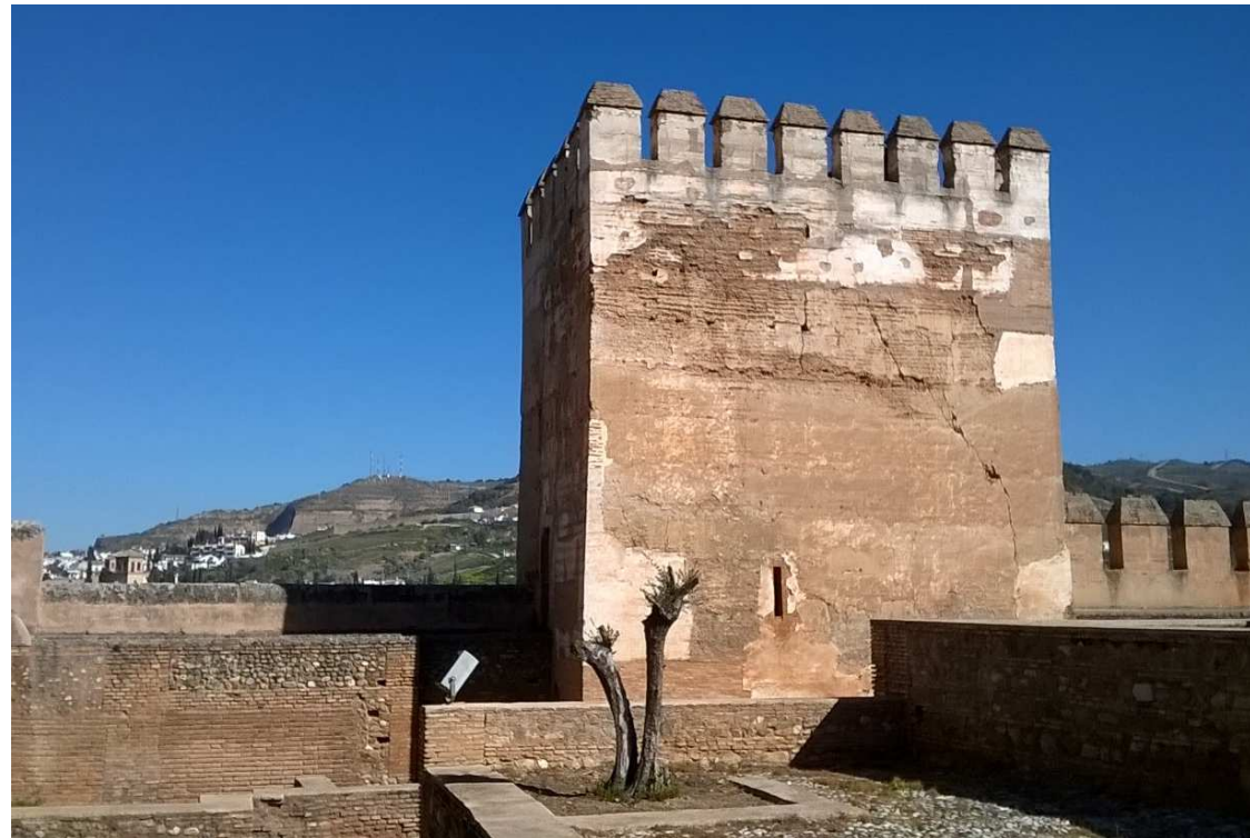
Restoration of walls and plasters in the Alhambra: «recognisability» through maintenance of all historic stratifications (photo: FC).
