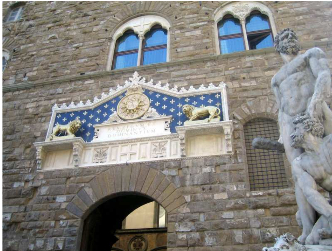
Florence, Palazzo Vecchio: use of high-tech windows resembling the original ones (source: Wikipedia).
