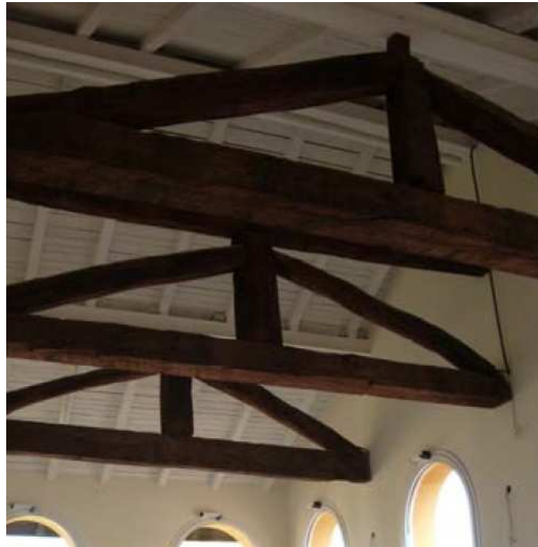
Restoration and re-use of original wooden trusses (source: nogap-progetti.com).
